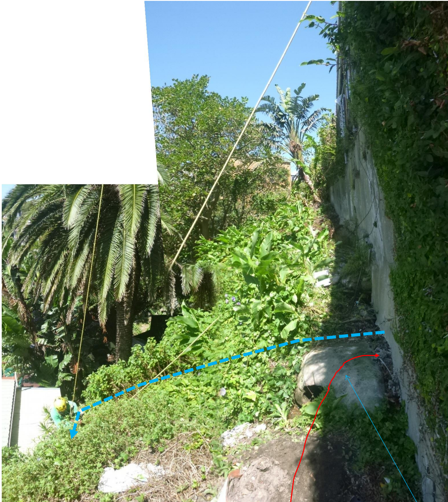
Photo 7. Cross Section 3 viewed towards the south-west. Note adjacent terrace wall has been cut down through detached sandstone block of the outcrop .
