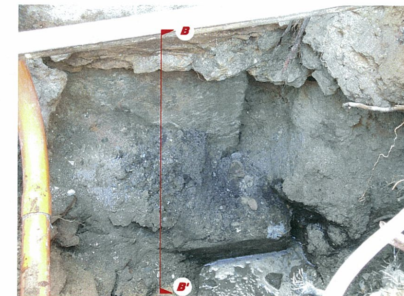
Photo 2: Showing corner of concrete footing
