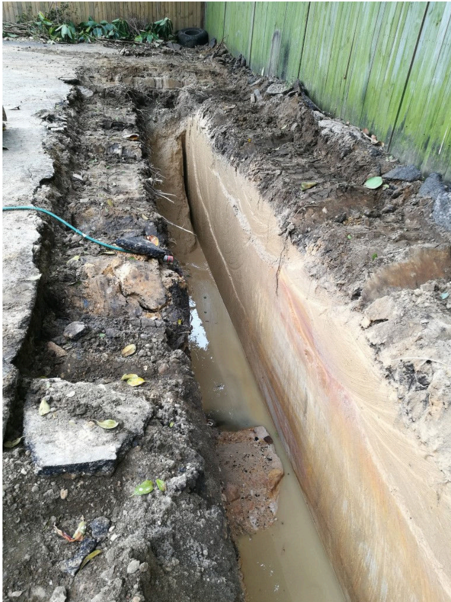
Historical Site Photograph of Sewer Diversion Trench, Photo 2 – View to west near Borehole BH3. Solid sandstone exposed at shallow depth along trench excavation.
