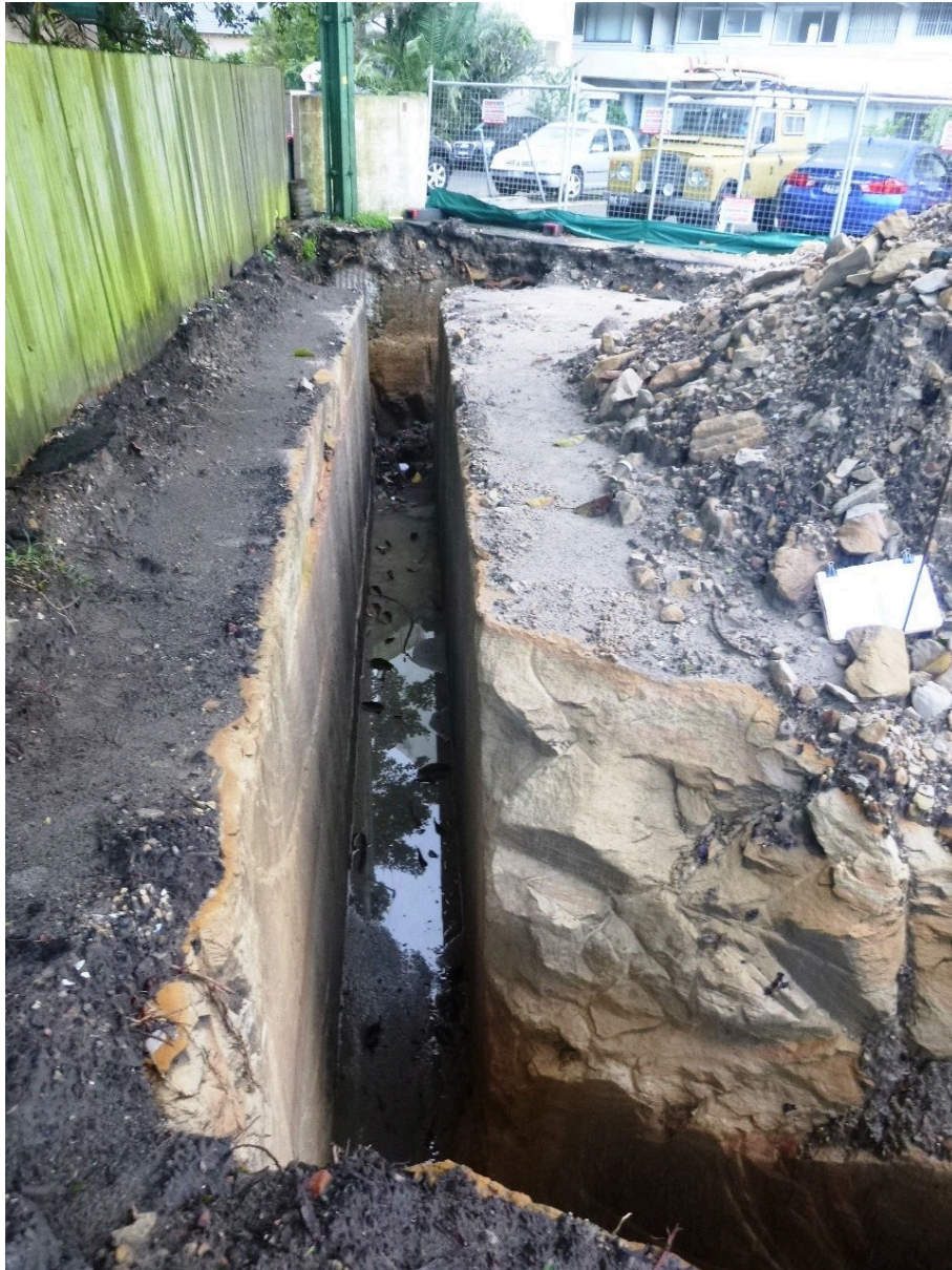
Historical Site Photograph of Sewer Diversion Trench, Photo 1 – View to east near Borehole BH3. Solid sandstone exposed at shallow depth along trench excavation.
