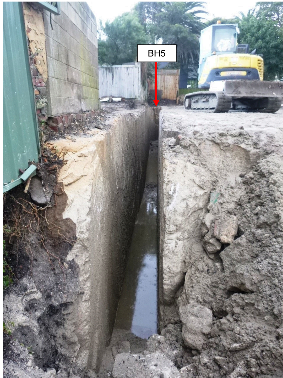
Historical Site Photograph of Sewer Diversion Trench, Photo 5 – View to north near Borehole BH101. Solid sandstone exposed at shallow depth along trench excavation. The approximate position of Borehole BH5 indicated as shown for reference.
