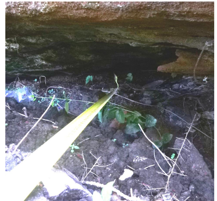
Photo 6. View into the weathered void.
