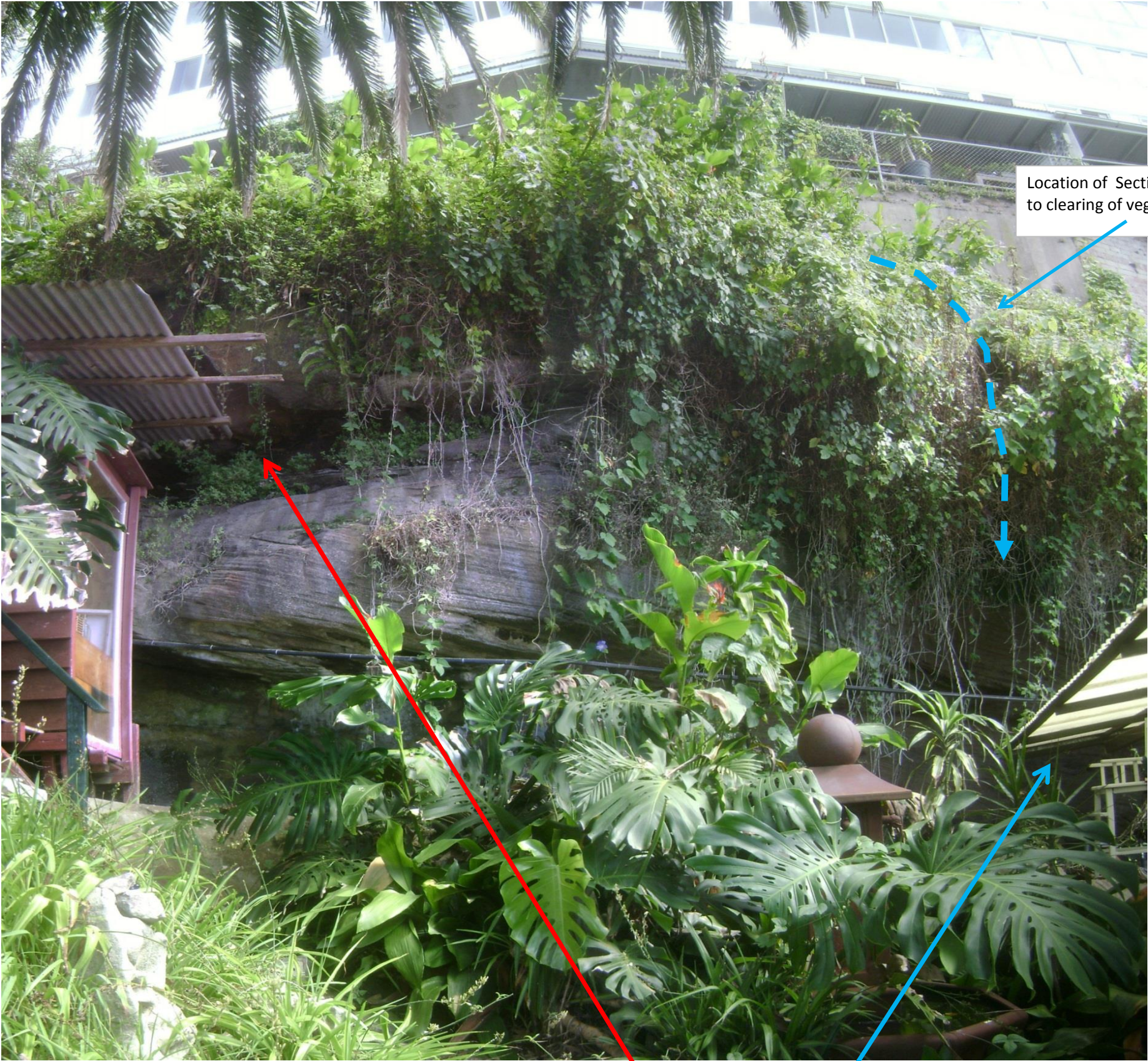
Photo 9. Area to the south-west of Section 3. Note higher level (of less extensive) undercut than the major undercut (refer to Drawing 2 to 4 photos) further to the north at Sections 1 to 3.
