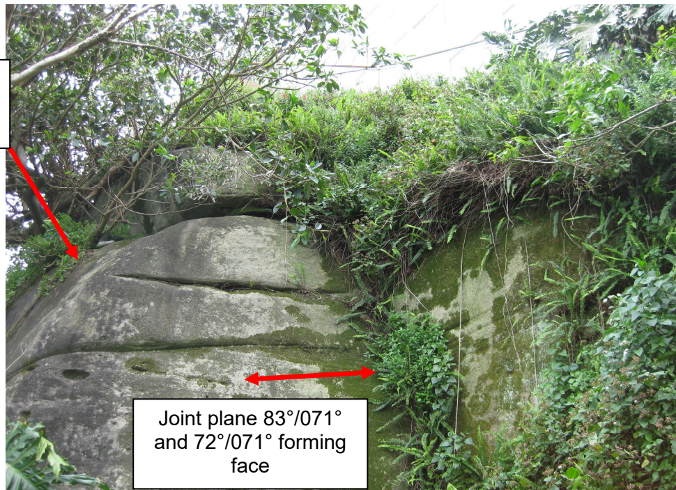
Mapping Traverse 105, Photo 6 – Side view of mapping traverse 105 (indicated). Persistent sub-vertical joint, forming a face, is indicated as shown.
